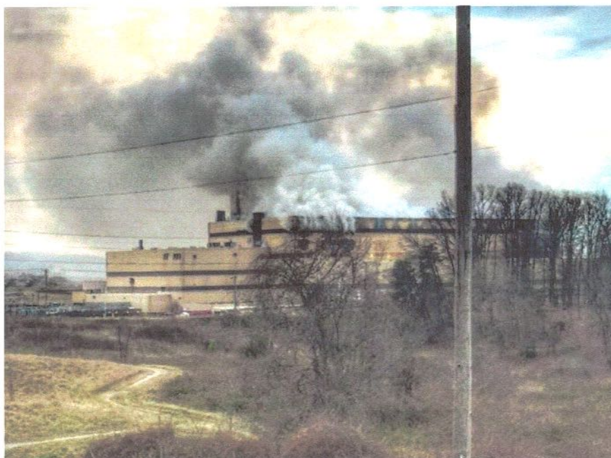
Covanta Fairfax County incinerator: Fire Feb., 2016 (938,000 tpa)
