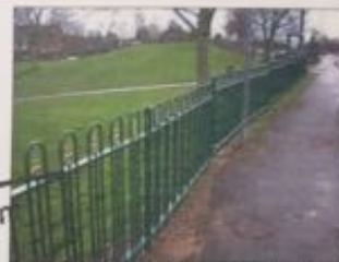
Sample of 2m High Railing to Western boundary
