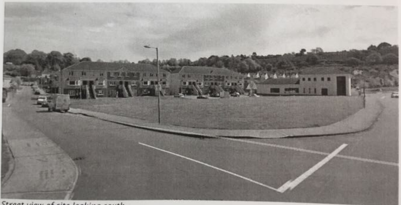
Street view of site looking south
