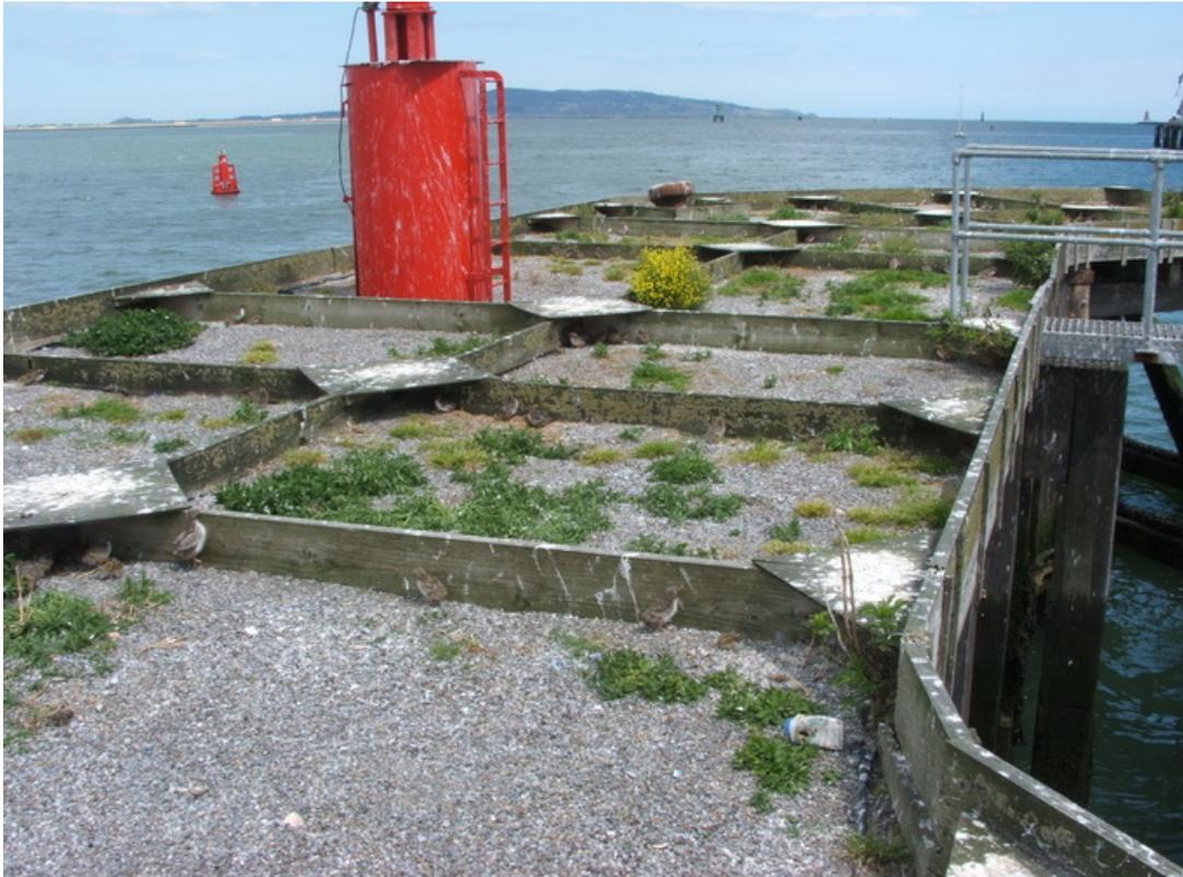
Plate 8: Wooden baffles with built-in shelter arrangement on former ESB dolphin at Dublin Port.
